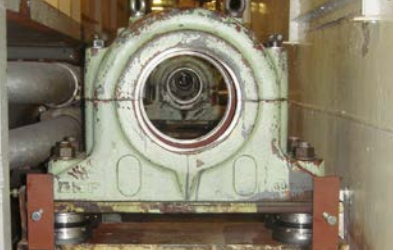
Intermediate shaft bearing Skid mounted diesel engine
